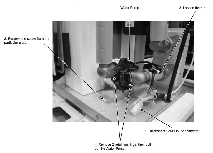
⚠ When reinstall the water pipe, use grease or water at the joining.
