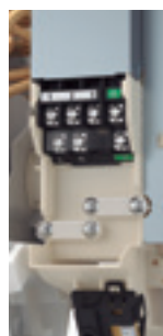
Bigger working space for wiring connection.
