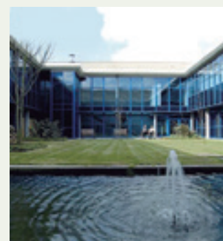
NHS Canford house clinic, Bournemouth, UK. VRF
