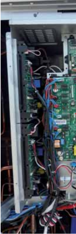
Binds a Comp wire by Holder wire.
