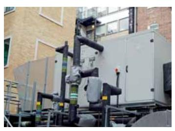
CONNECTION TO CHILLED WATER COILS IN AIR HANDLING EQUIPMENT. AIR HANDLING APPLICATION
